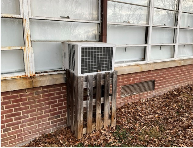
25 - TYPICAL THRU-WINDOW UNIT
