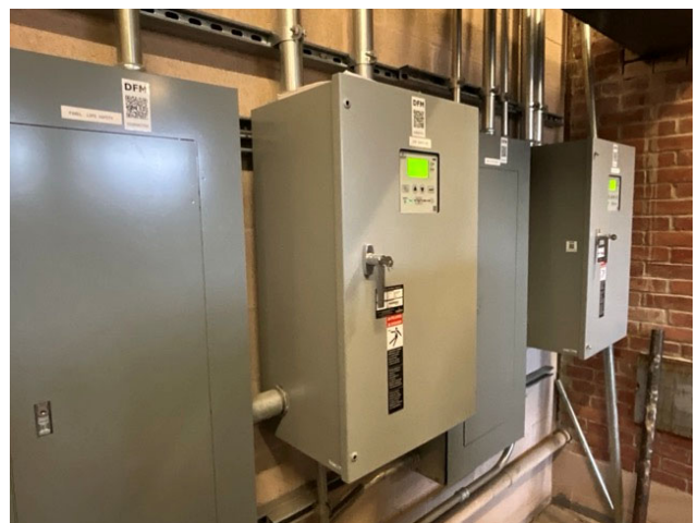
18 - AUTOMATIC TRANSFER SWITCHES
