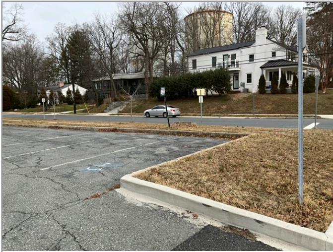
OVERVIEW OF ACCESSIBLE PARKING AREA
